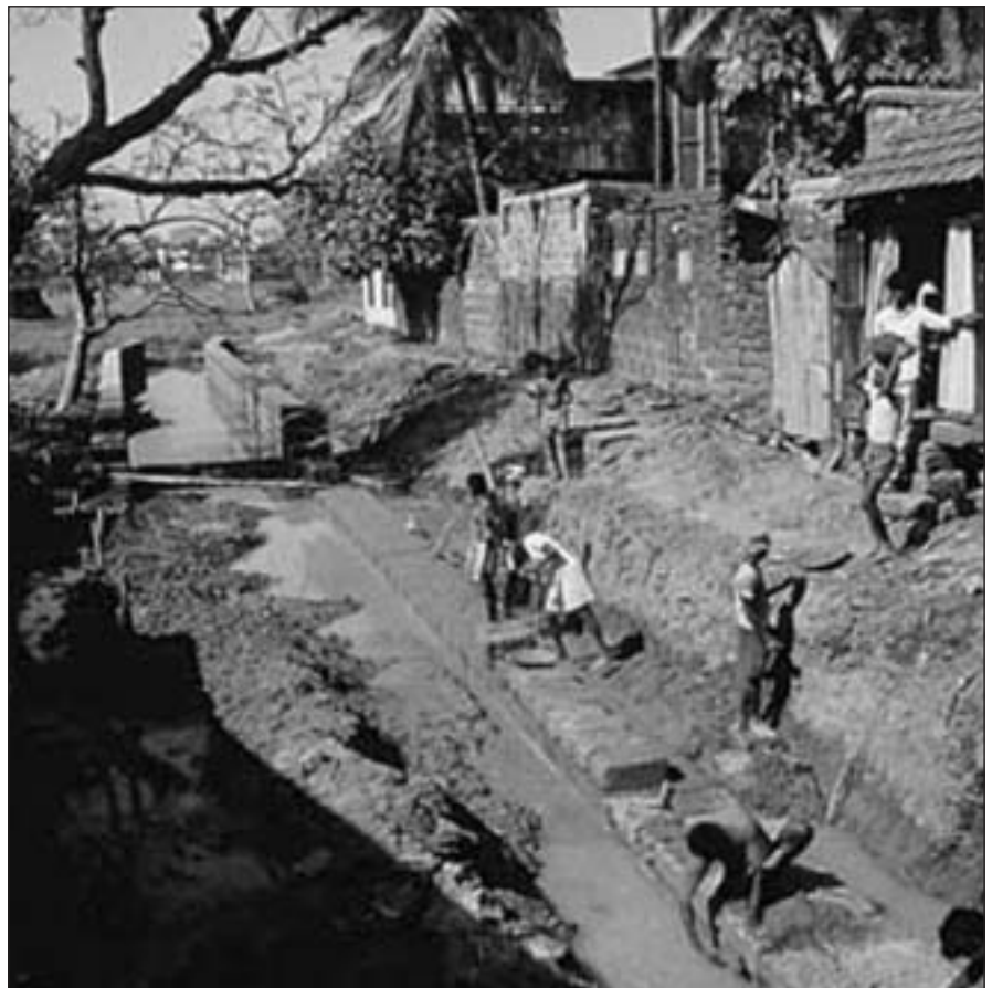
Community construction flood storm drainage chan
