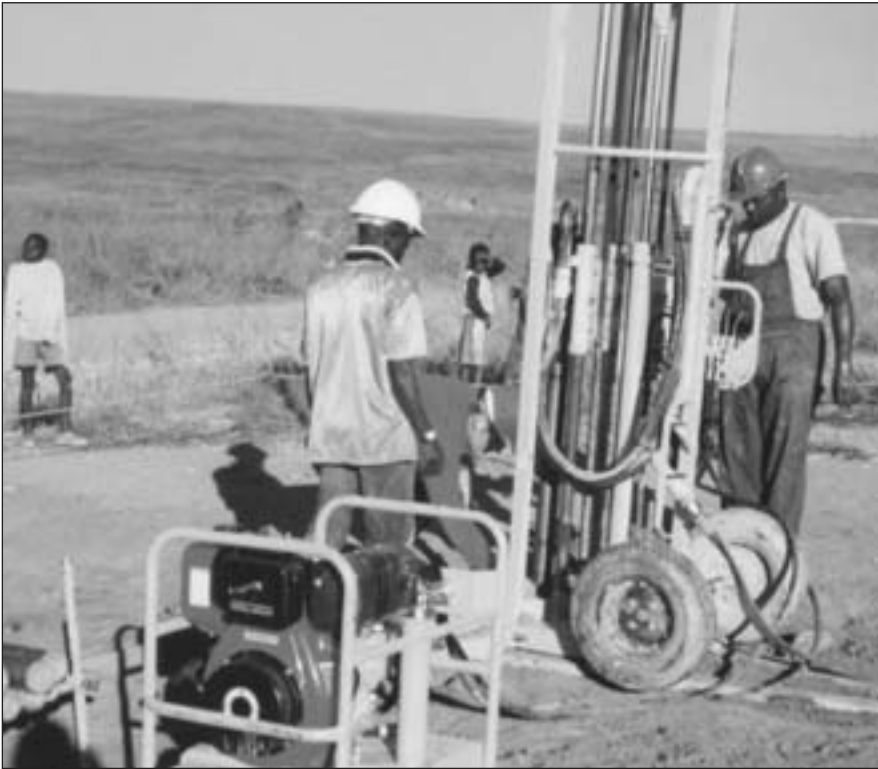
Drilling of a borehole for community water supply project WEDC
