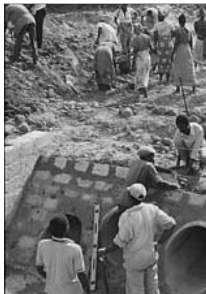
Community participation of road culvert, WEDC
