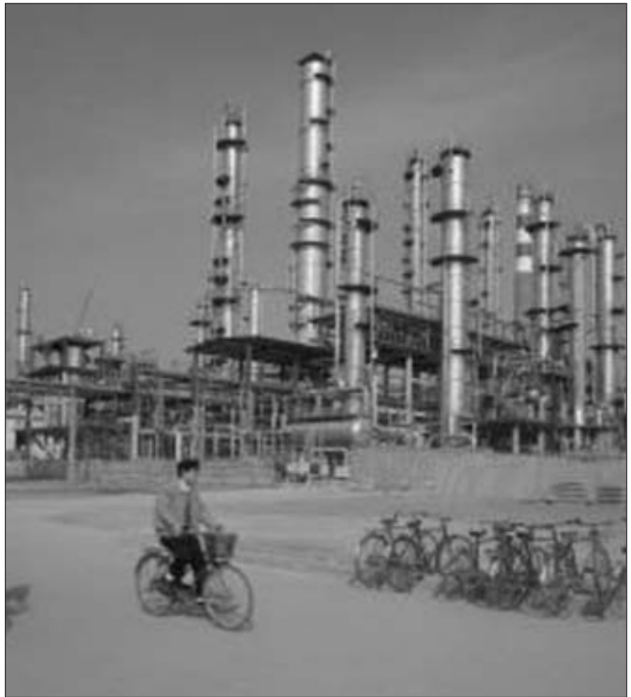
Gas processing plant, Malampaya Project, Philippines
